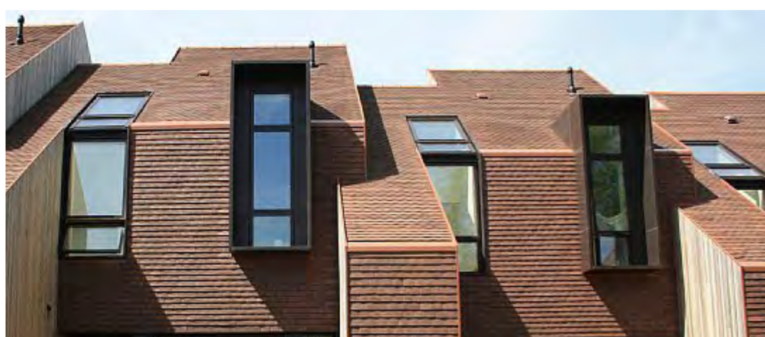
Feature dormer windows are a dominant feature of the Golden Mede development facing the proposed Sixth Form Centre
