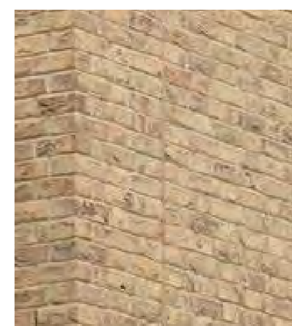
Light brickwork to match school brickwork
