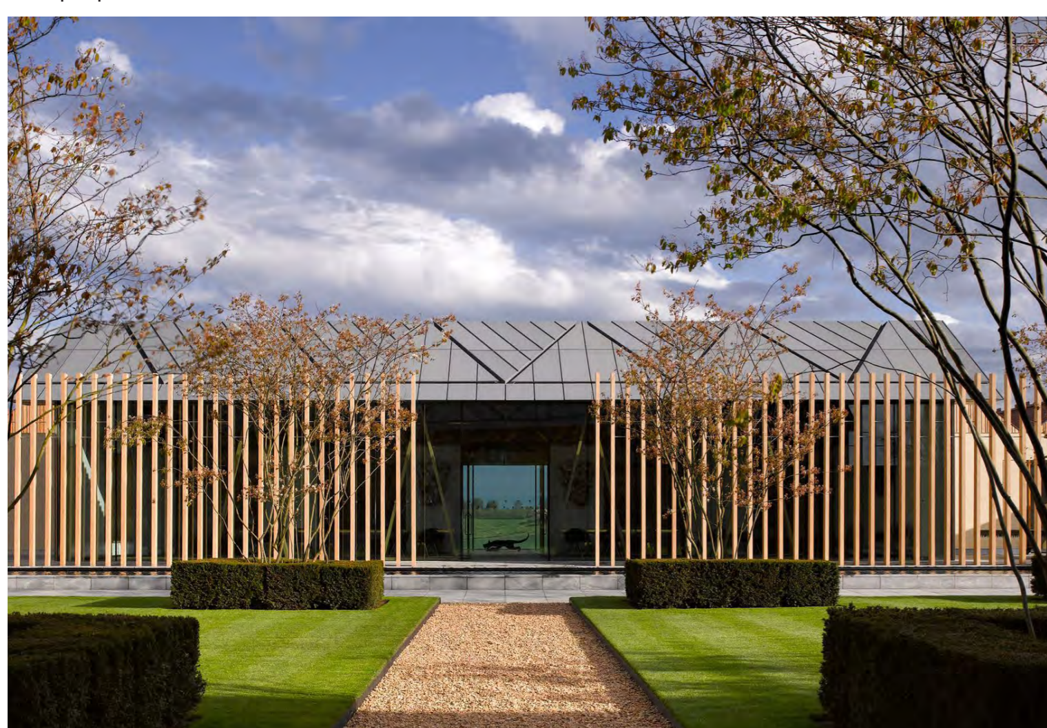
Vertical timber louvres are referenced around the auditorium and on the south elevation
